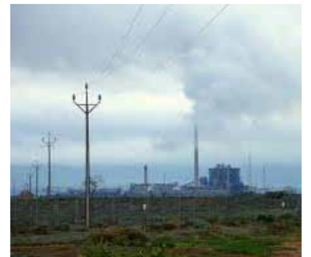
Port Augusta Power station
