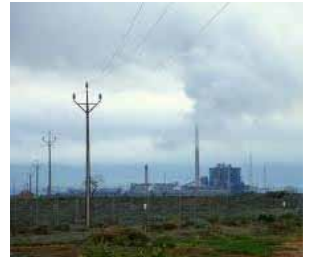
Port Augusta Power station
